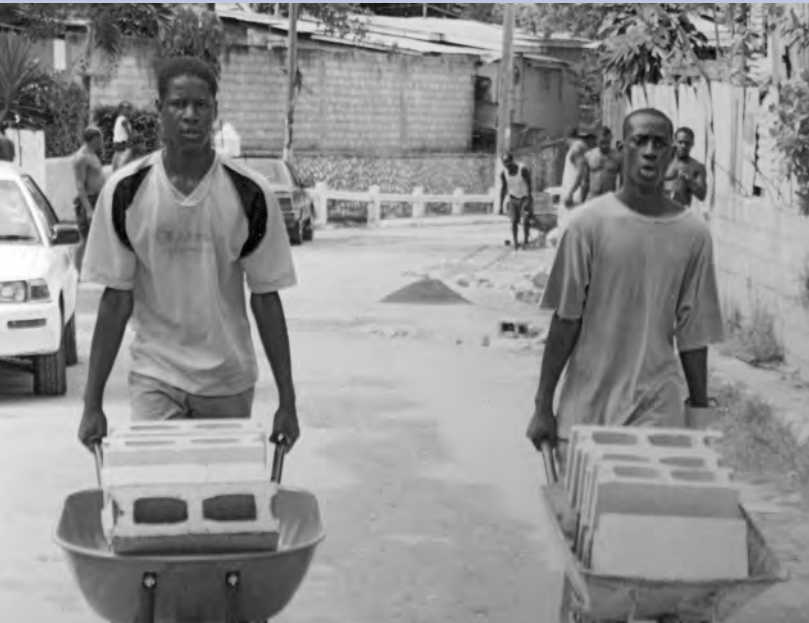
BELOW: Grants Pen residents help haul cinder blocks during a community clean-up project in 2004.
